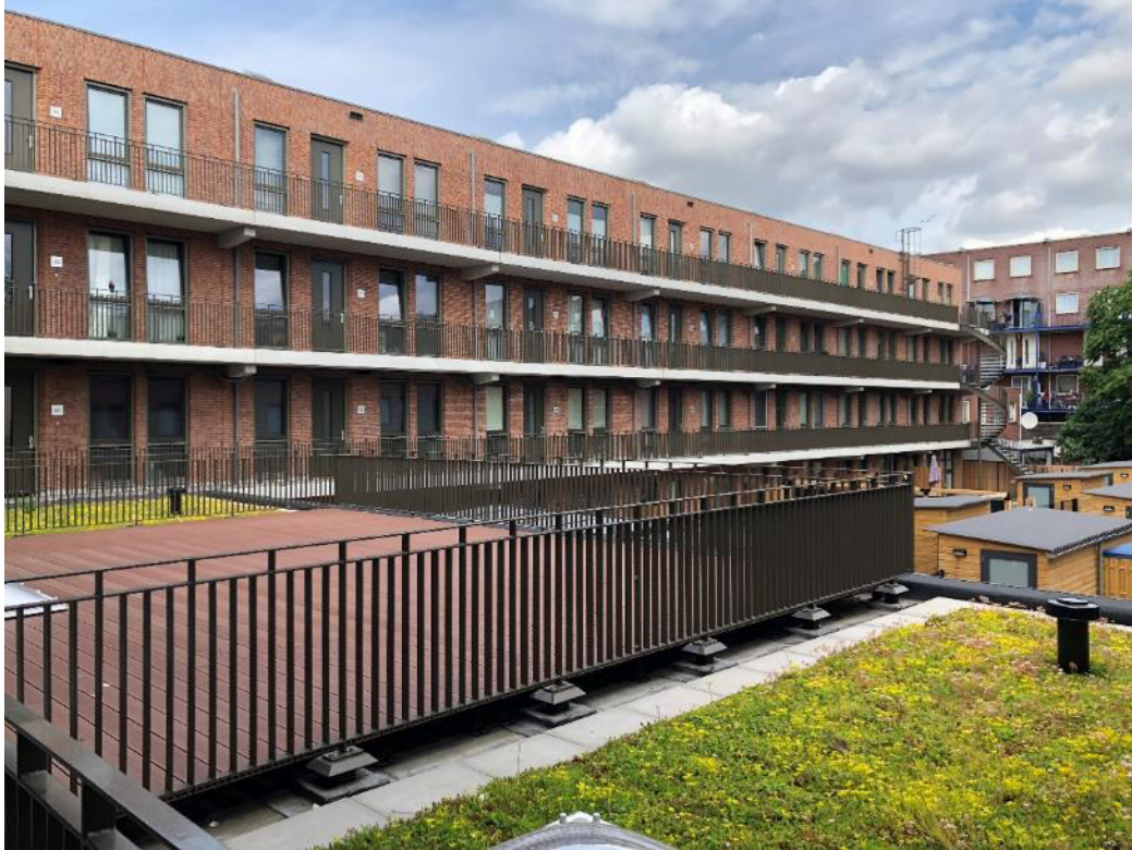
Access to upper-level apartments through interior courtyard with gallery entrances. This layout is particularly cost-effective because circulation space is primarily outdoors.
