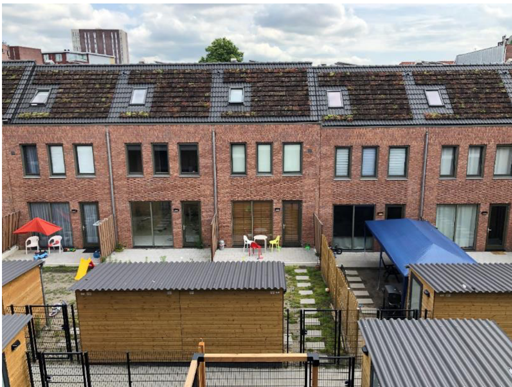
View of single-family row houses is taken from the complex's interior courtyard. Shows private storage sheds and flood-mitigating green roof system.
