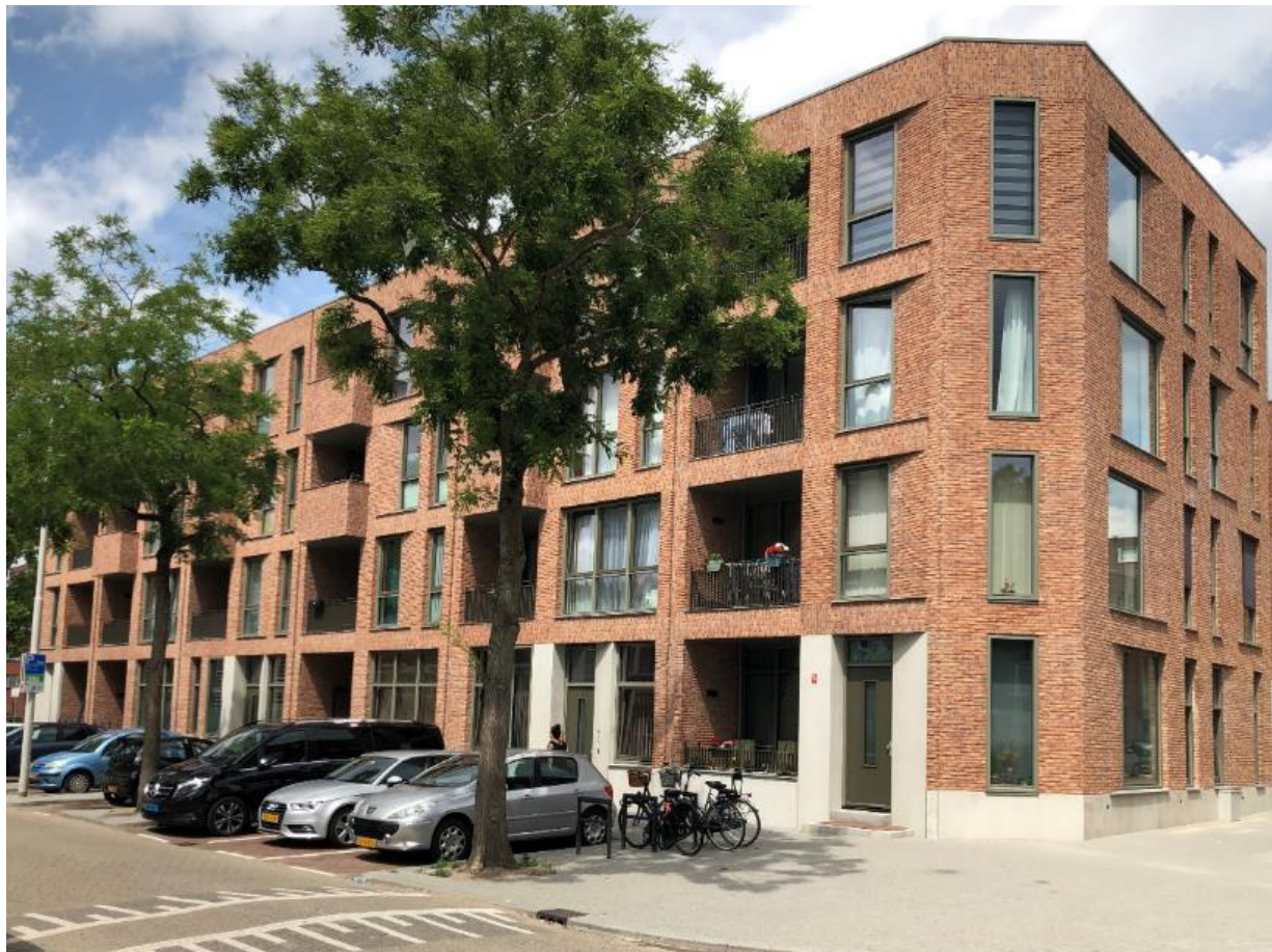
Exterior view of the Rotterdam Architecture prize-winning project Malieklos by Woonstad Rotterdam. Malieklos is a €12.5 million development with 51 apartments and 33 single-family row houses, all of them social housing units with rents below the liberalization threshold of €763. All photos by author unless otherwise noted.
